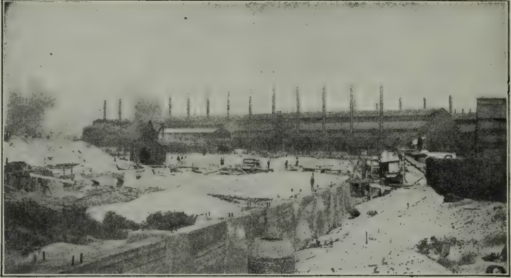
Gary, Indiana, when under construction.
